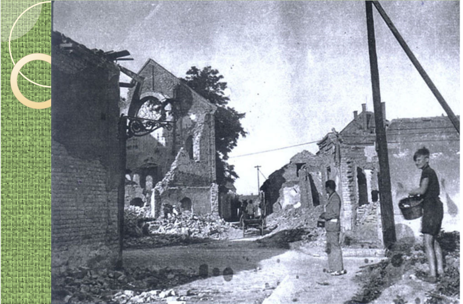
the destroyed streets
